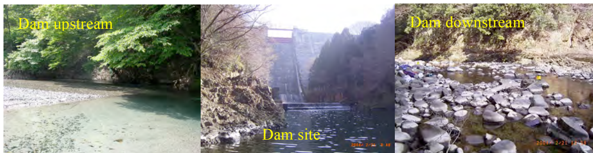
Figure 1. Comparison of the riverbed landscape between upstream and downstream reaches of the Yasugawa Dam in the Yasu River in central Japan. The dam is as old as 53 years and the distinctive riverbed armoring can be observed. White part of rocks indicates thick accumulation of organic matter originated from the reservoir.
